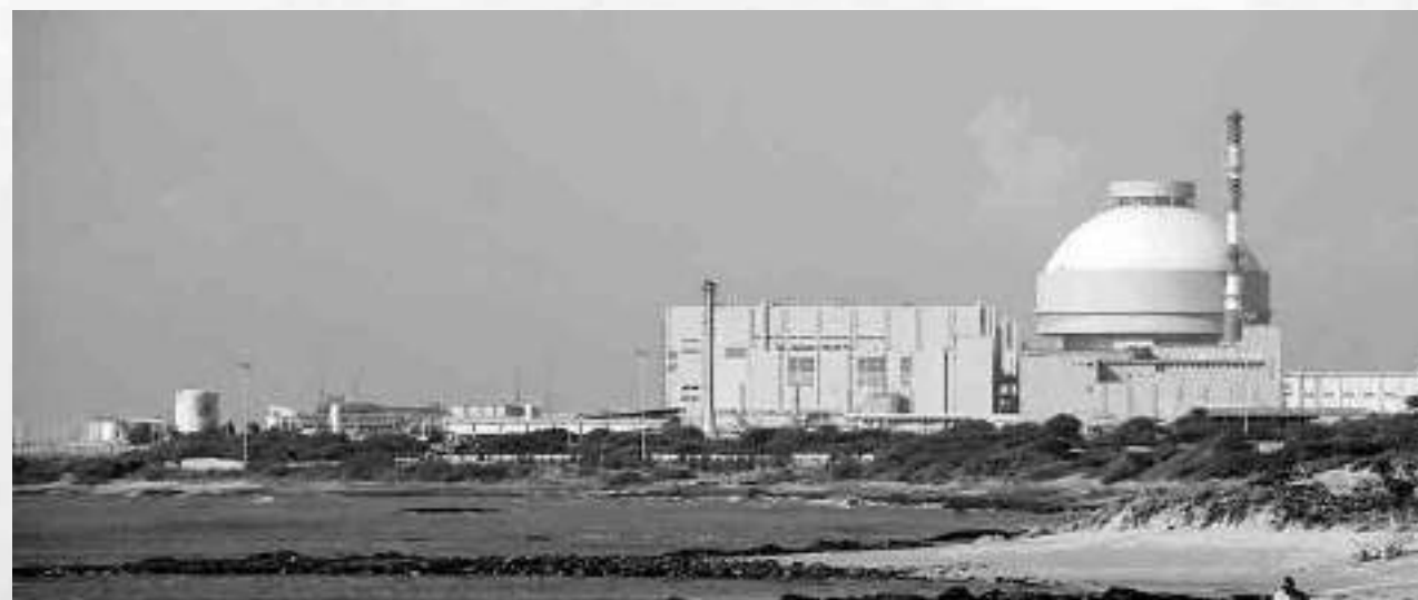
Kudankulam nuclear power plant – India's largest nuclear power station
